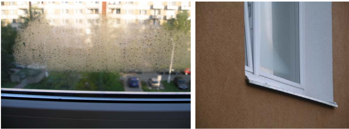
Figure 5: Glass of a new window, non-transparent thanks to the condensation of water
