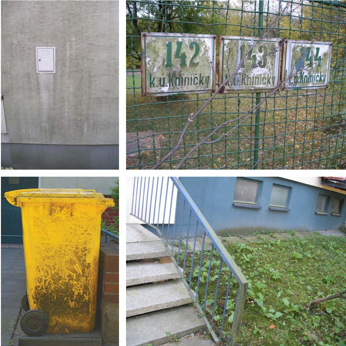
Figure 3: Attack of algae observed on various structures and equipments in the city
